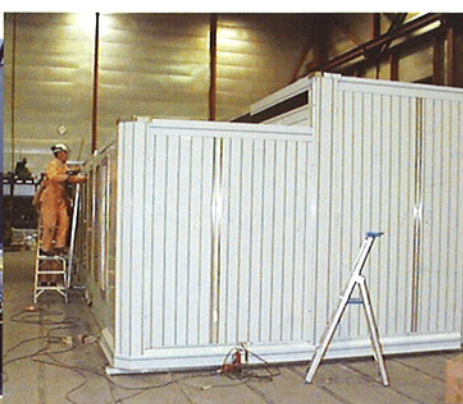
STATFJORD A - HEALTH CENTRE TEST ASSEMBLY OF FLAT PACK DELIVERY
