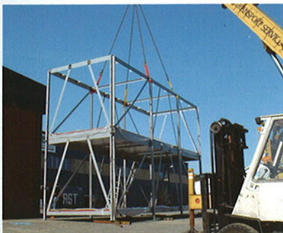
STRUCTURAL ASSEMBLY OF OFFICE MODULES LB 4000
