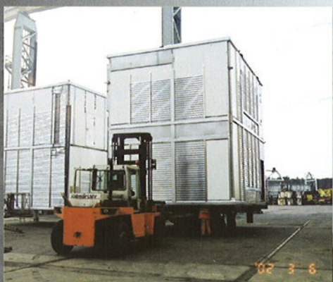
VALHALL WHP MODULES - LOADOUT
