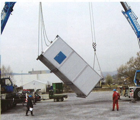
TESTLIFTING OF STATFJORD A - CONTROL ROOM MODULE
