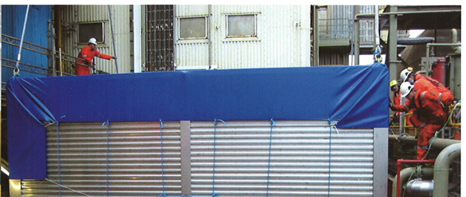
4 STOREY OFFICE BLOCK INSTALLED DECK BY DECK ON STATFJORD A
