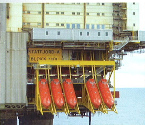
STATFJORD A MODULES AFTER INSTALLATION
